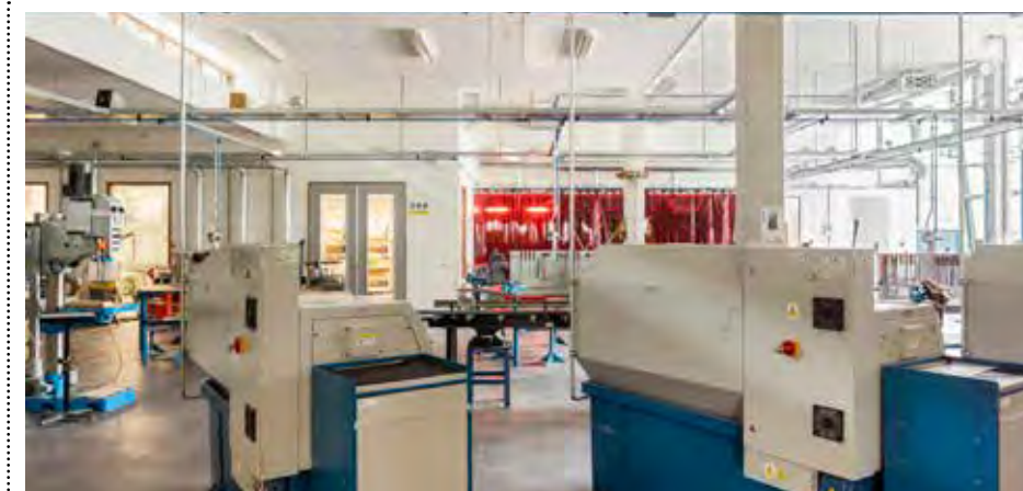
Heraklith A2 Wood Wool was installed in Da Vinci College in the Netherlands to minimise noise from adjoining classrooms
