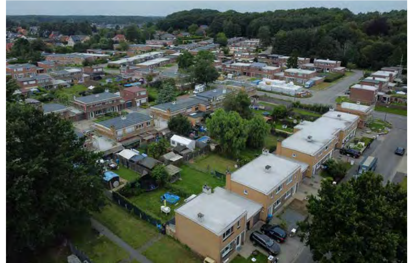
Work begins in Aarschot on the second biggest Knauf Energy Solutions initiative in Belgium
