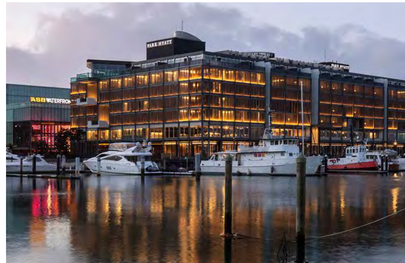
The Park Hyatt Hotel in Auckland, New Zealand , features Earthwool in internal partitions and on external walls
