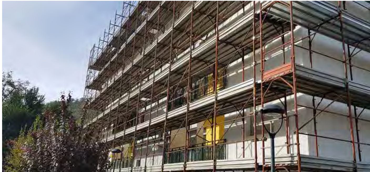
Knauf Insulation's SmartWall S C1 is installed in social homes in Italy's Salerno province: our Italian team is supporting a digital platform to improve building energy efficiency
