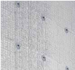
Arrangement of the weld pins
