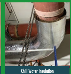
Chill Water Insulation
