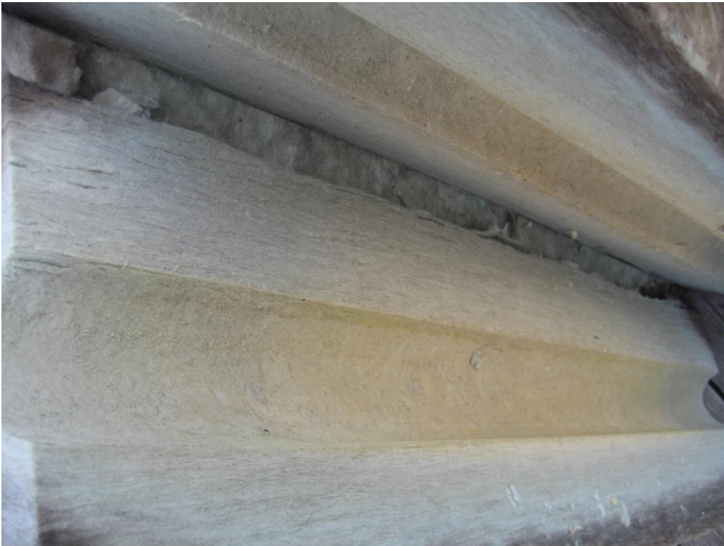
Figure 2. Layer 1 After Testing
