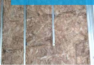
Knauf Insulation was engaged to provide products, which would help to meet or exceed the acoustic and fire-resistant requirements for this project. Knauf Insulation Acoustic batt 14kg/m³ was installed to double stud metal framed walls, in addition to fire rated plasterboard to achieve high performance outcomes and help create a sealed intertenancy envelope.
