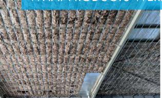
The entire ceiling was battened to create a cavity for the insulation. Earthwool® ceiling batt, R5.0 was installed in combination with a pliable building membrane to achieve high thermal performance, low emissivity and a highly durable finish. The walls required a particularly high R-Value of R4.0, this is 38% higher than the minimum standard of insulation used in external walls in Melbourne (standard is R2.5).
