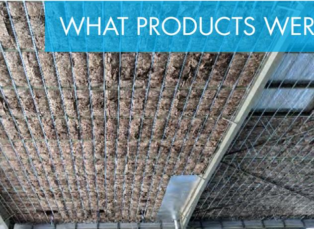
The entire ceiling was battened to create a cavity for the insulation. Earthwool® ceiling batt, R5.0 was installed in combination with a pliable building membrane to achieve high thermal performance, low emissivity and a highly durable finish. The walls required a particularly high R-Value of R4.0, this is 38% higher than the minimum standard of insulation used in external walls in Melbourne (standard is R2.5).
