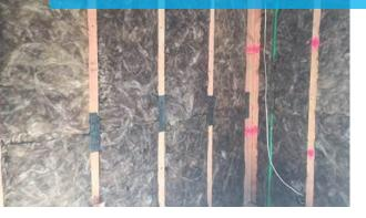
Due to limited space in the internal wall cavity, the thickness of the insulation was crucial. The insulation needed to fit inside the cavity without compression and it was imperative it provided superior thermal and acoustic performance.
