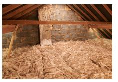
If you want to add additional layers, these should be laid in parallel to the second layer (not crosslaid). Fit any additional layers at the same time as the second layer, so you can continue to use your crawl boards across your joists.
