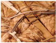
If you're unsure whether your cables are appropriately sized for their load, speak to an electrician. If in doubt, always rest cables on top of insulation.
