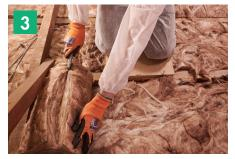
**Remember:** don't insulate directly beneath a water tank and make sure any cables under a high electrical load are resting on top of your insulation.
