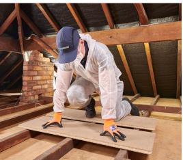
Lay crawl boards across the joists, ensuring they're supported by three joists – you'll use these to safely move around the loft space, without putting your foot through the ceiling!
