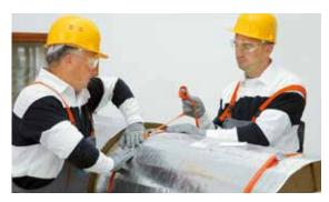
The pipe-shell will be temporarly held by tension belts or rubber straps to ease final fixing.
