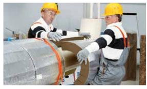
Separate two step mounting of custom-fitted pipe segments (each segment covering 180° of the circumference).
