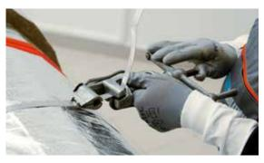
In the last step the pipe segments need to be fixed with metal straps. Please consider national norms with regards to dimensioning.
