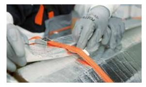
Longitudinal seams are closed with alu straps and circular seams are sealed with standard alu tape (recommended width:= min 50mm).
