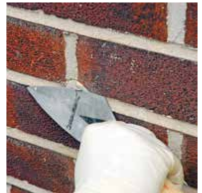
3. The holes are repointed with mortar
