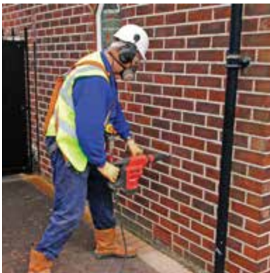
1. A series of 20mm holes are drilled in the mortar lines
