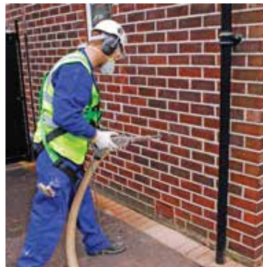
2. Supafil CarbonPlus is blown into the cavity
